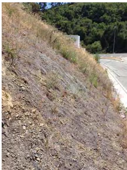
Photo 11: Cut slope at the junction of Edmonds Road and Edgewood Road composed of disintegrated sandstone and shale
