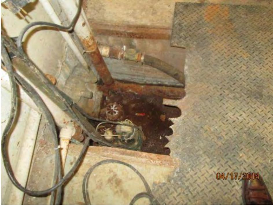
**Photo P-5 - Sump Pumps in Trench**
