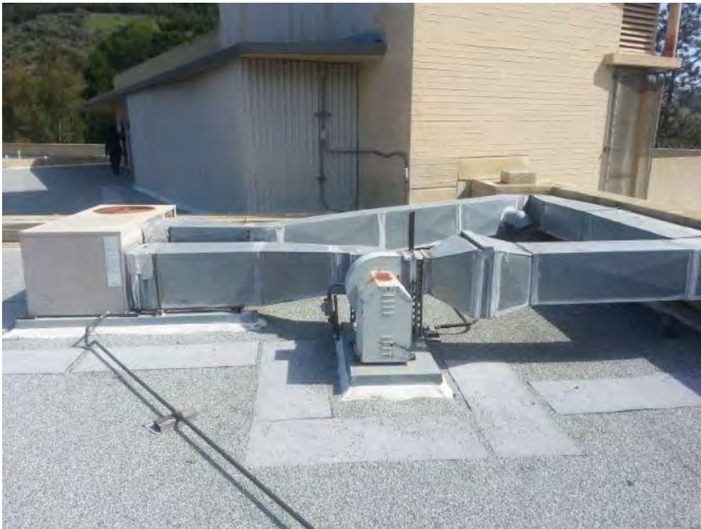
**Photo M-9 – Roof Packaged Heat Pumps**
