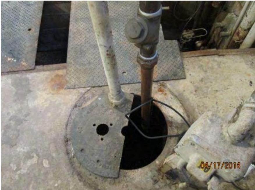
**Photo P-4 - Sump Pit in Boiler Room**
