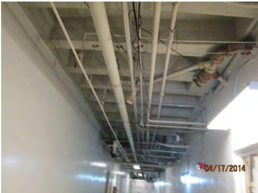
**Photo P-2 - Hub & Spigot Cast Iron Piping**
